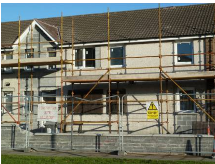
Photo Multi-element improvement work in Westwinds estate, Newtownards
