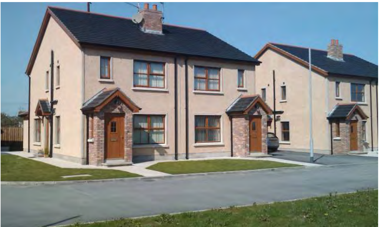
New Build Scheme – Eglish Road, Eglish (Rural HA)
