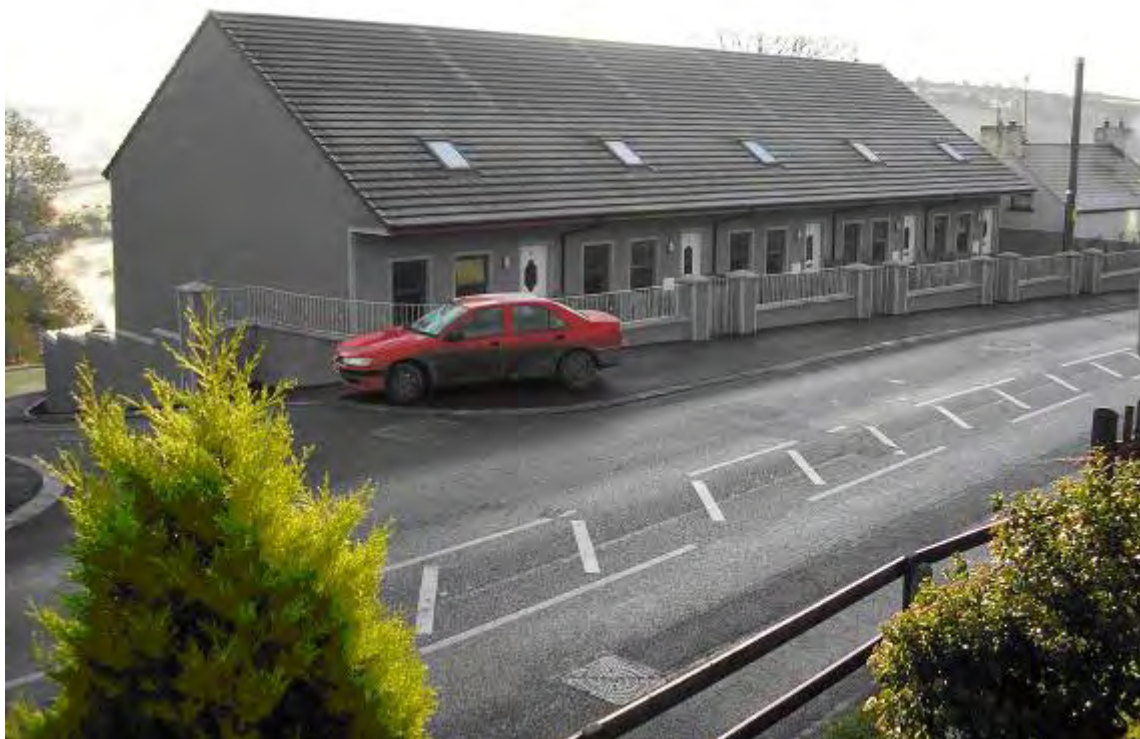
New Build Scheme – 1-5 Fedorna Heights, Poyntzpass (Oaklee HA)
