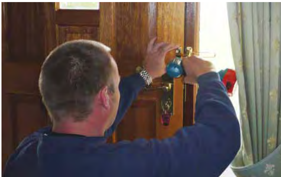
Security Door Bar being fitted
