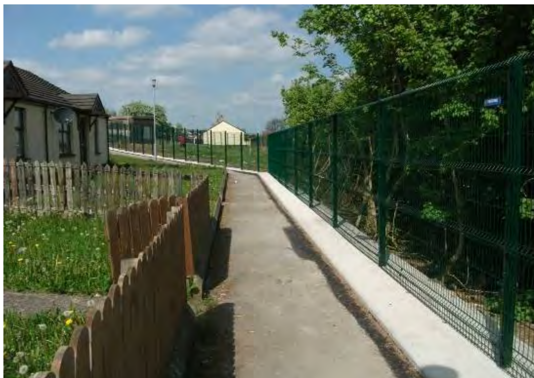
Fencing erected at Mullacreevie Park, Armagh City
