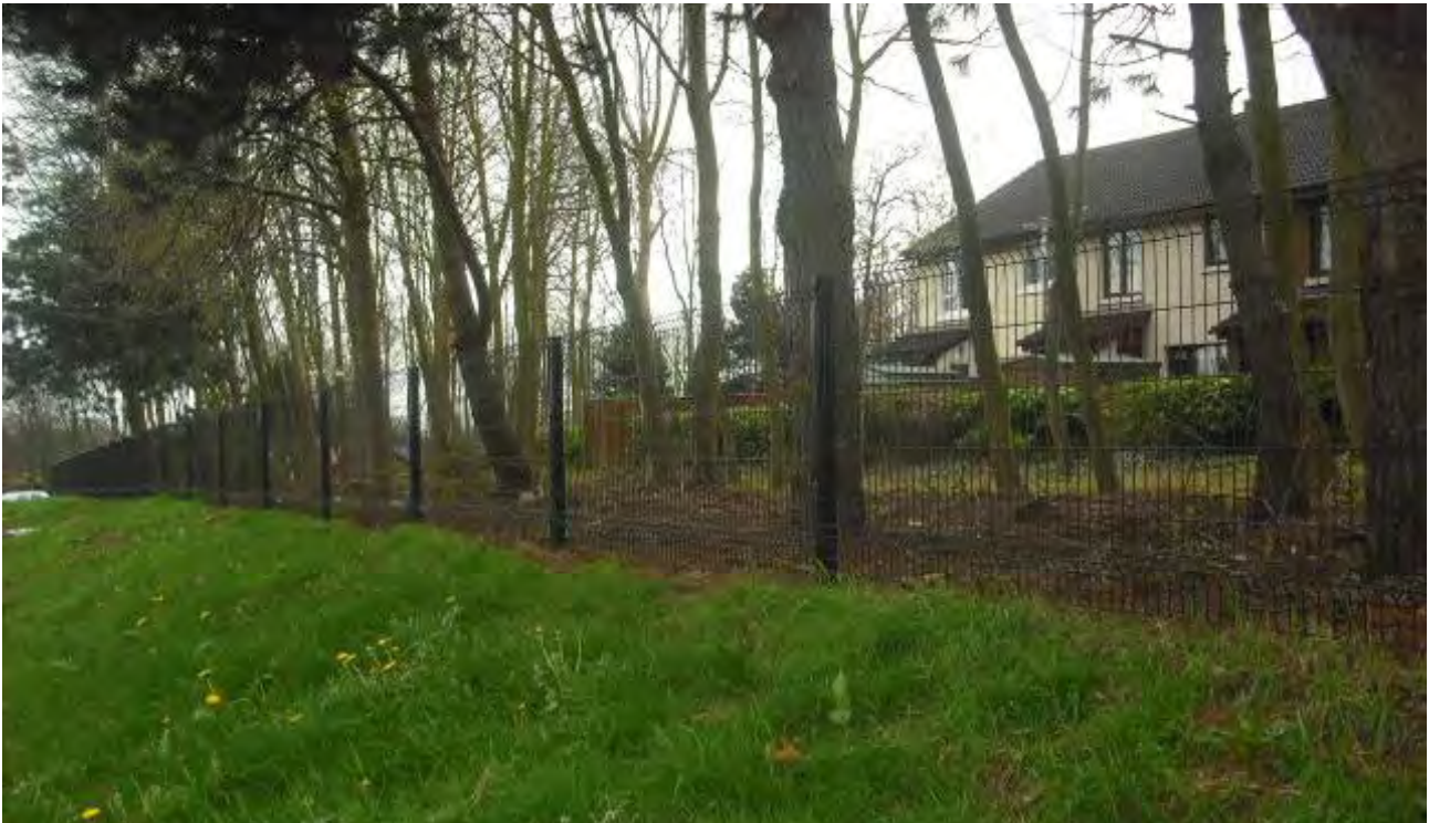
New Fencing at Prince William/Knockmore Road
