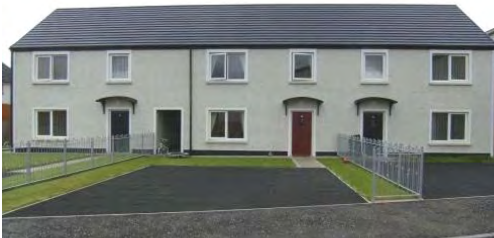
New social housing development at Scutchers Lane, Draperstown
