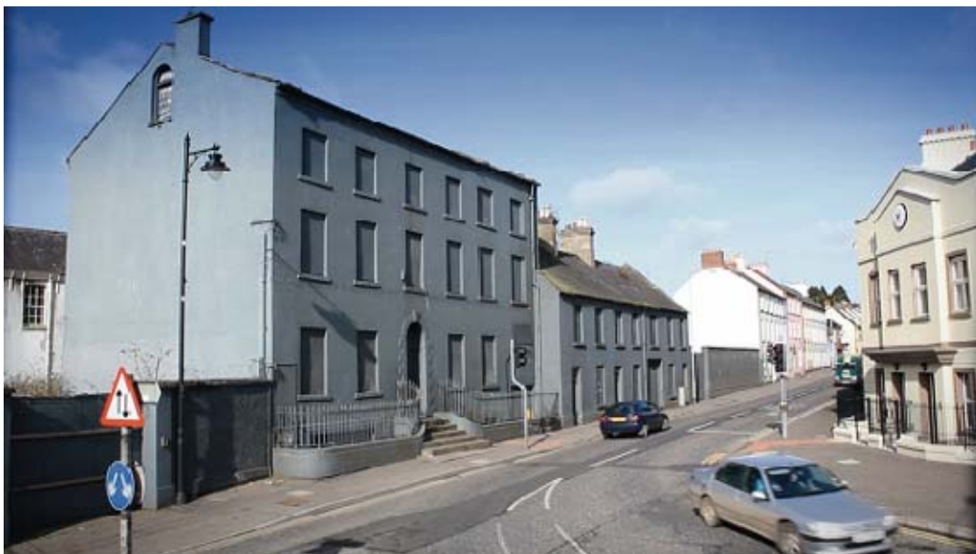
Canal Street Phase 4 area – Before redevelopment
