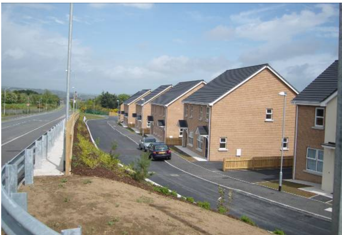
New Build Scheme – Demesne, Carnagat (South Ulster HA)
