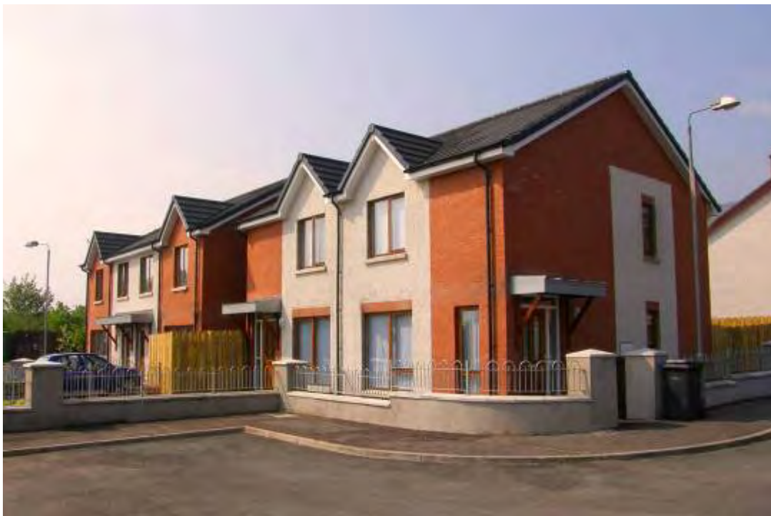
New build scheme at Bawnmore developed by Habinteg Housing Association
