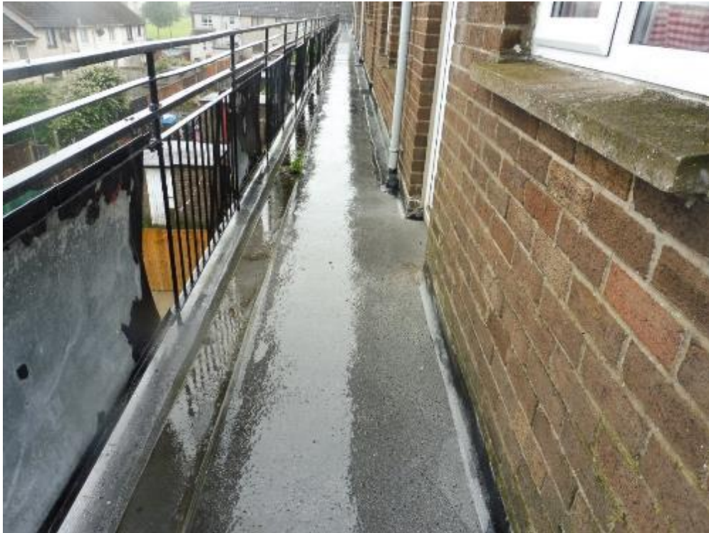
Figure 21 Asphalt to concrete balconies
