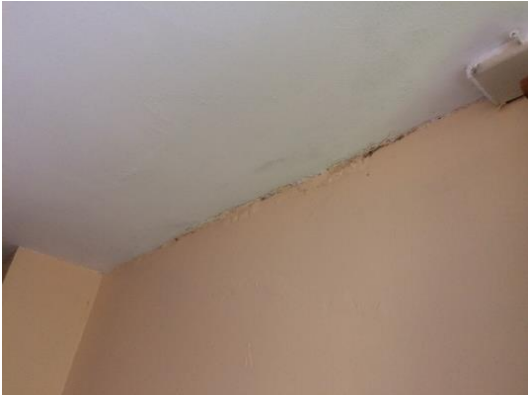
Figure 27 Evidence of water penetration to bedroom at [REDACTED]
