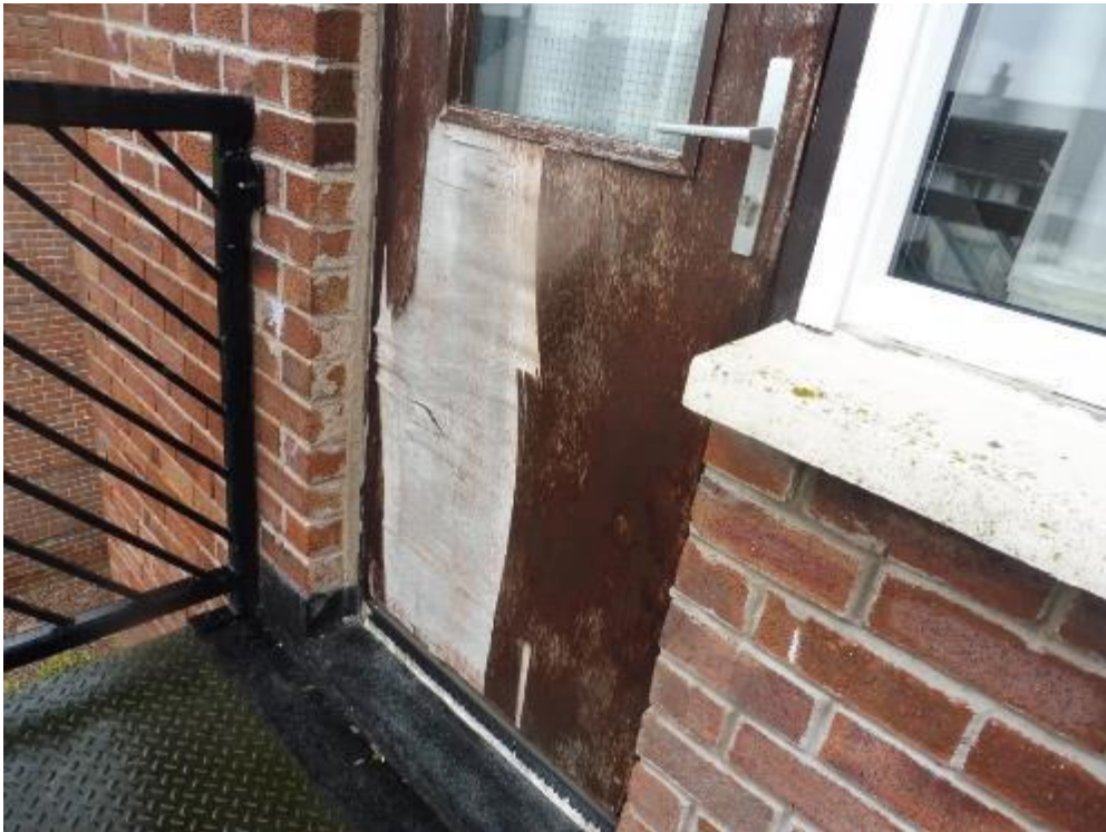
Figure 30 Rear fire exit door in need of replacement
