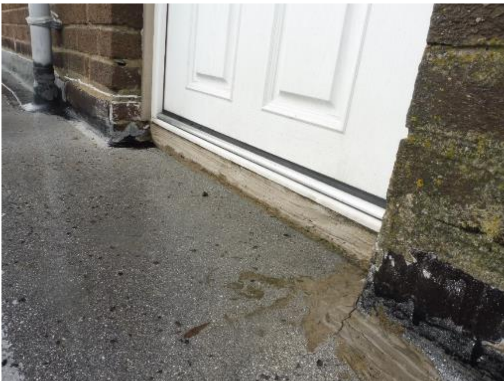
Figure 24 Where new doors have been installed, no asphalt upstand provided
