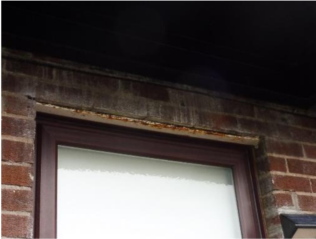
Figure 17 Steel angle irons affected by rust
