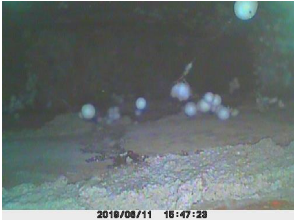
Figure 15 Rossmore Green - Void in insulation
