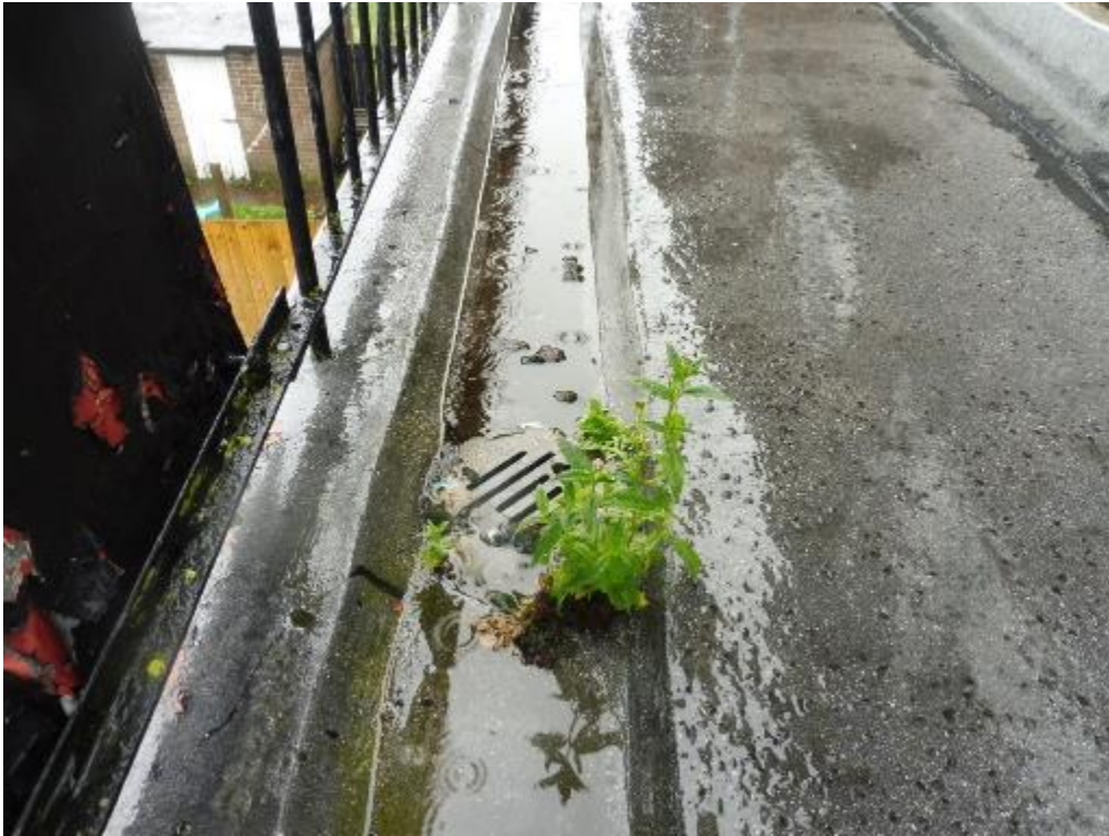
Figure 25 Outlet from the balcony to downpipe below
