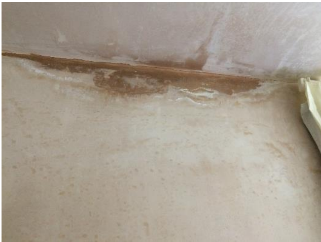
Figure 26 Water staining to rear external wall to bedroom at [REDACTED]
