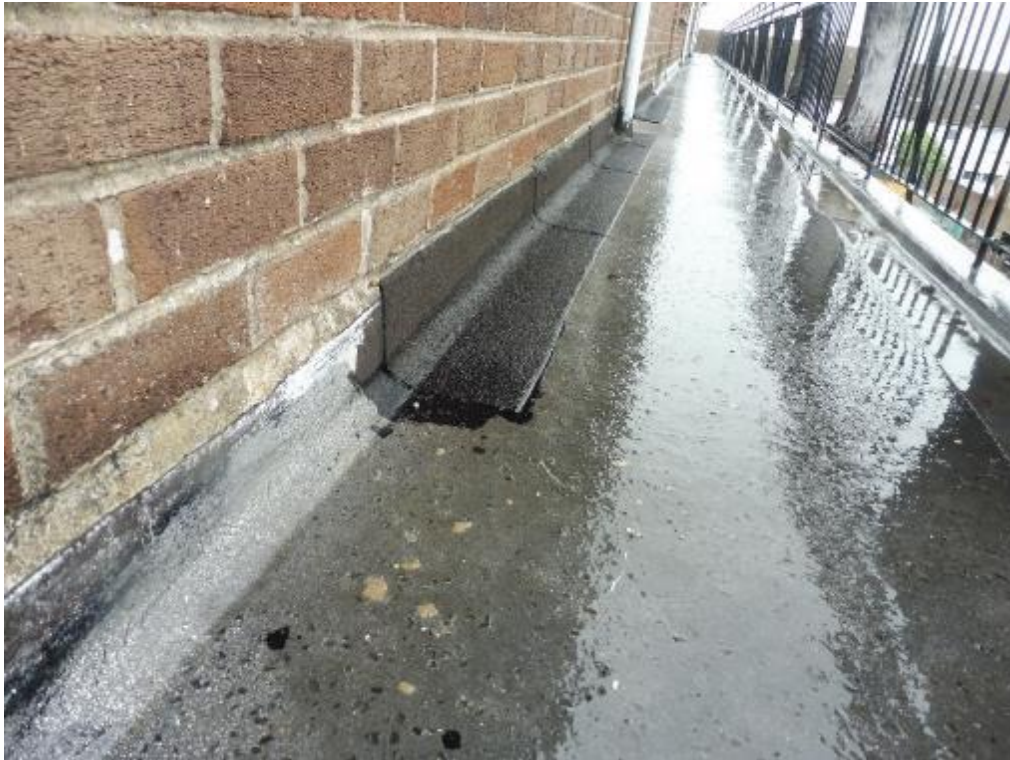
Figure 23 Repairs carried out to where the asphalt meets the external walls at flats
