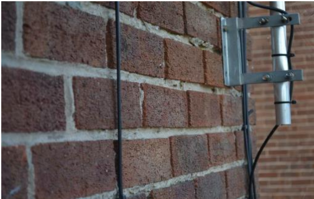
Figure 16 Poor mortar pointing to the existing brickwork
