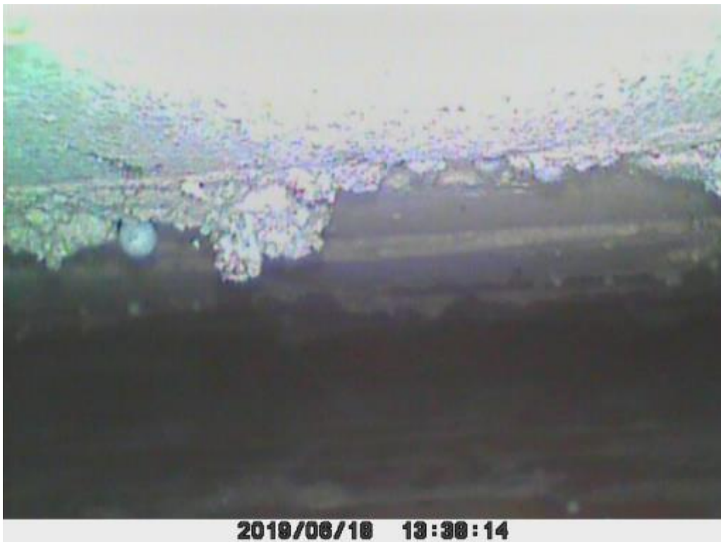
Figure 14 [REDACTED] – Glassillan Grove – Insulation absent
