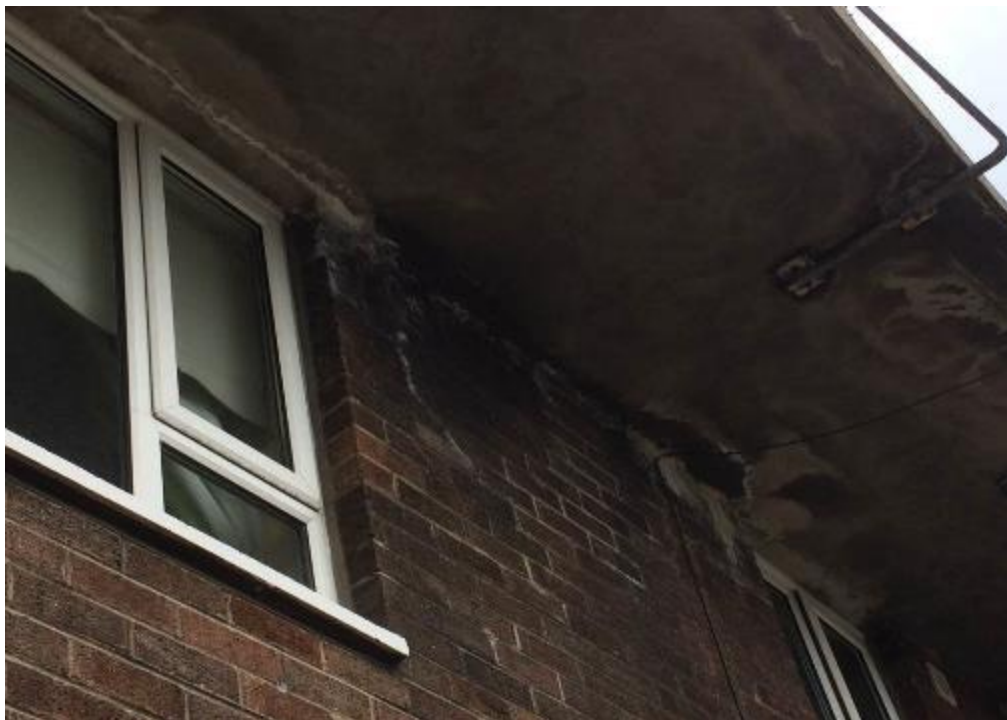
Figure 22 water staining to underside of concrete balcony and external walls of maisonettes
