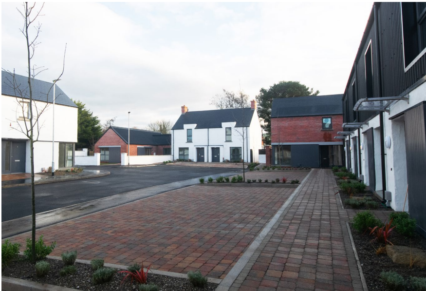
Old Mill Court, Sion Mills. Rural Housing Association
