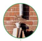
possible causes: insufficient drop in qutter
