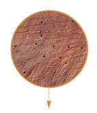
what is wrong: holes in timber or 'powdery' woodwork
