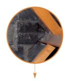
what is wrong: damp chimney stack or dampness on underside of slates
