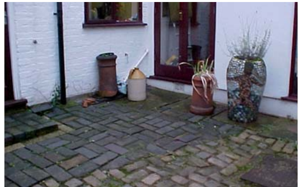
Figure 13: Examples of Category 1 hazards for falls on the level – the uneven and slippery cobbles, combined with a raised manhole cover and numerous small steps, significantly increase the risk of a fall
