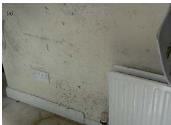
Figure 20: Damp and mould growth
