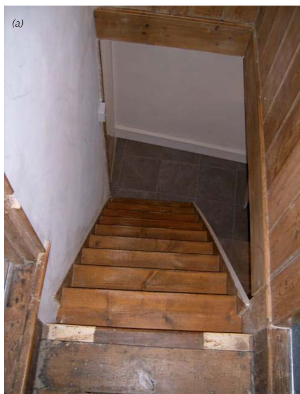
Figure 12: Examples of Category 1 hazards for falls associated with stairs and steps (a) Steep internal stairs, with trip step at the top and no handrails (b) External steps with sloping nosings, covered in slippery algae
