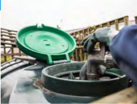
**A**n oil spillage can occur due to accidental damage, a leak to your oil tank, oil line or boiler or due to tilting or propping up your tank. You may notice a strong smell of oil, staining on hard surfaces, discoloration of grassed or planted areas and/or visible damage to oil appliances.
