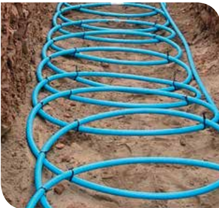
Installing ground source heat pump pipes.
