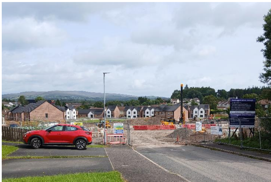
Coolnagard, Omagh, being developed by Choice Housing Association, which is currently onsite. Phase 1 provided 26 units, 12 two-bedroom houses, 12 three-bedroom houses, one 4-bedroom wheelchair bungalow and one 5-bedroom wheelchair bungalow. Phase 2a will provide 21 units, 13 two-bedroom houses, 6 three-bedroom houses, one 3-bedroom wheelchair bungalow and one 4-bedroom wheelchair bungalow
