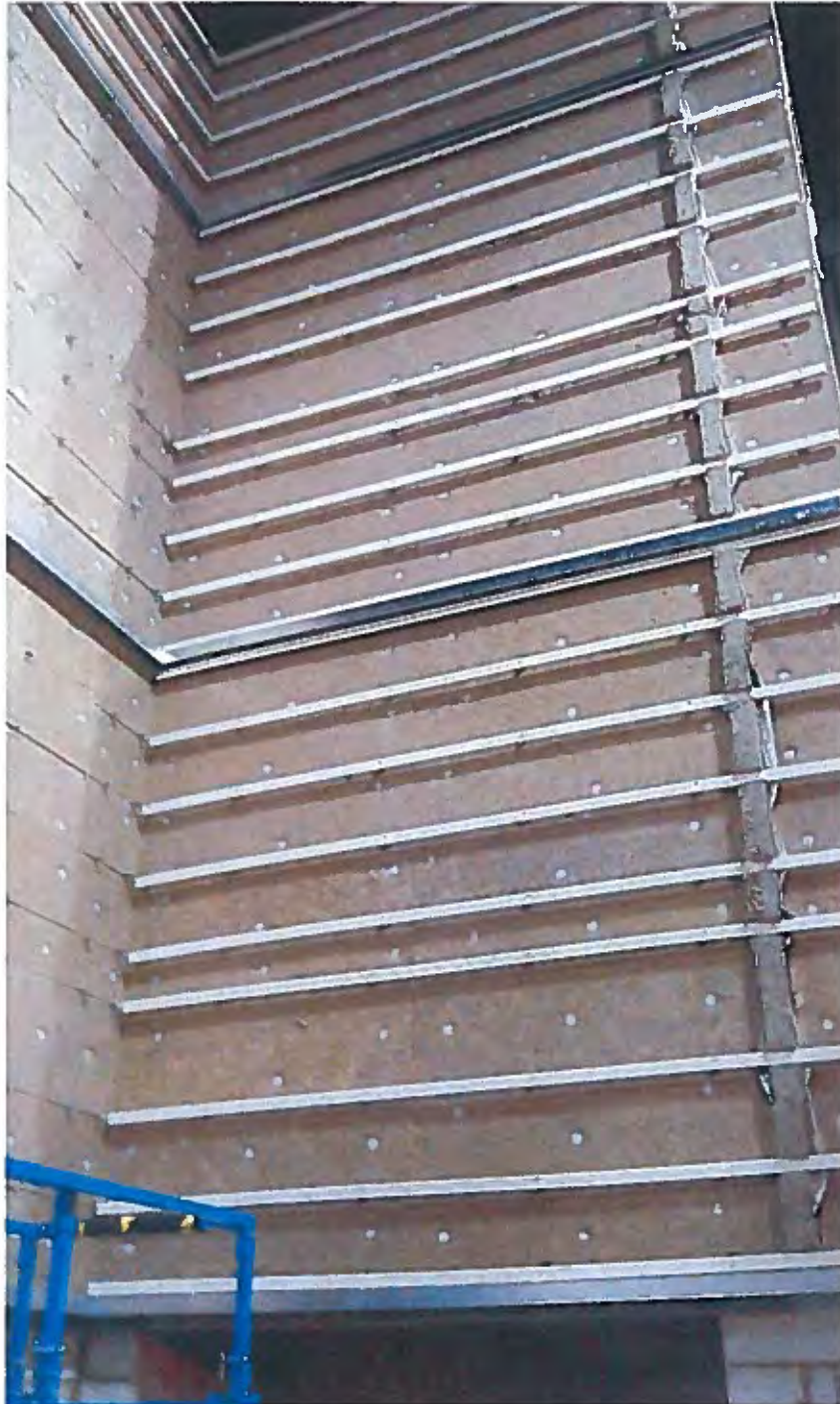
Figure 1. Photograph of the system during construction – Insulation, Cladding rails, horizontal and vertical fire breaks
