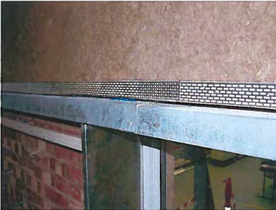
Figure 15 Galvanised steel flashing above the window.
