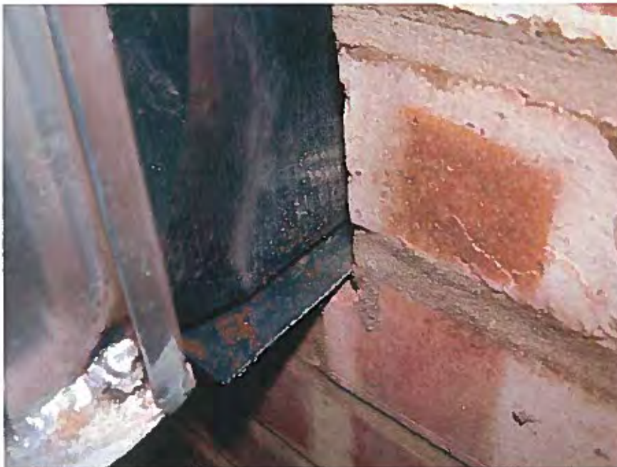
Figure 14 Brickwork adjacent to window assembly was dry.
