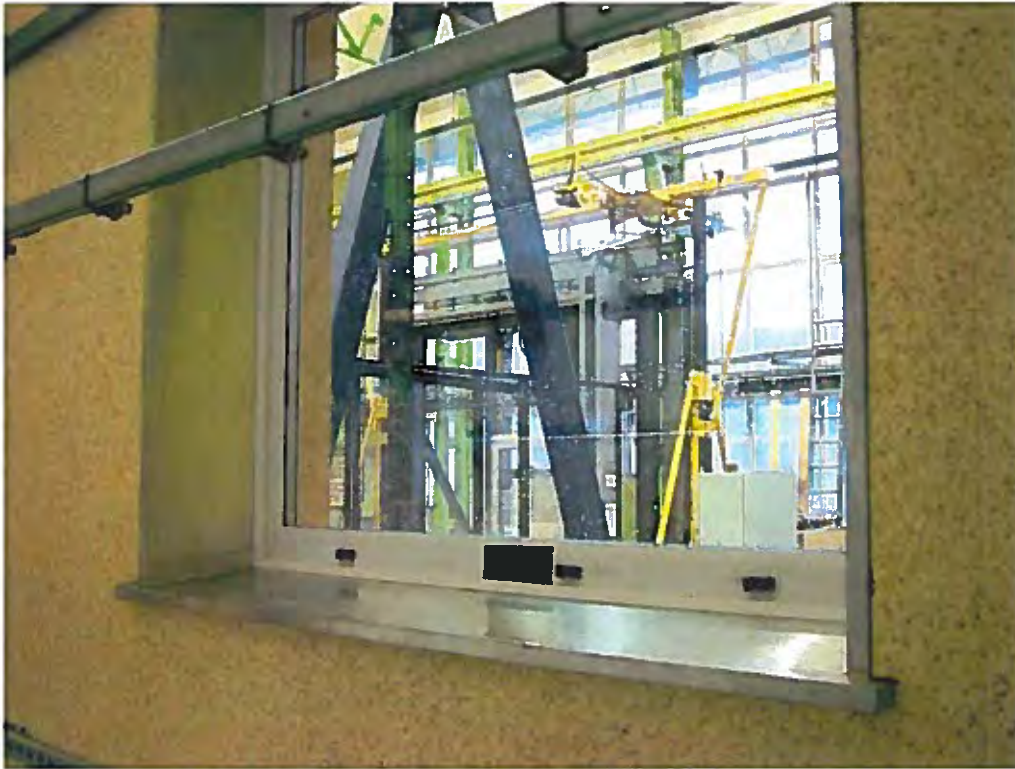
Figure 10 Window assembly installed in backing wall.
