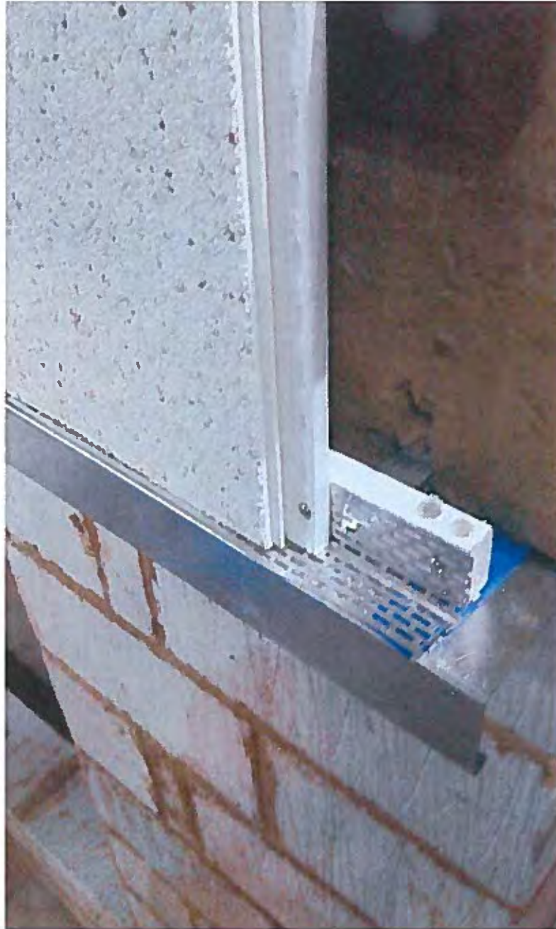
Figure 3. Photograph of the system during construction – insulation layer, bottom rail and Vinylit bottom vent fixing detail.
