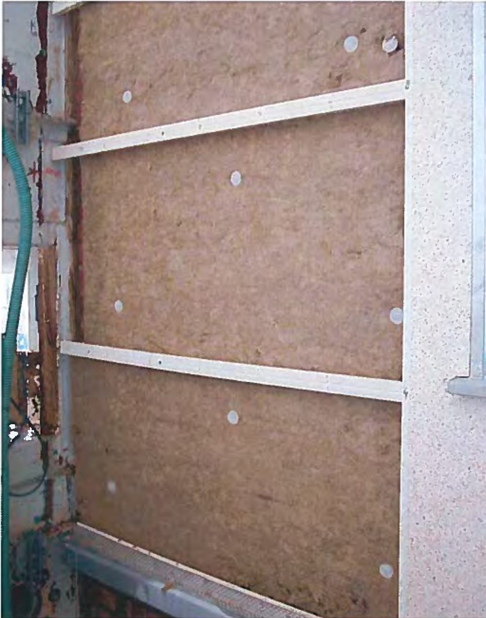
Figure 12 Rainscreen panels partially removed showing the insulation.
