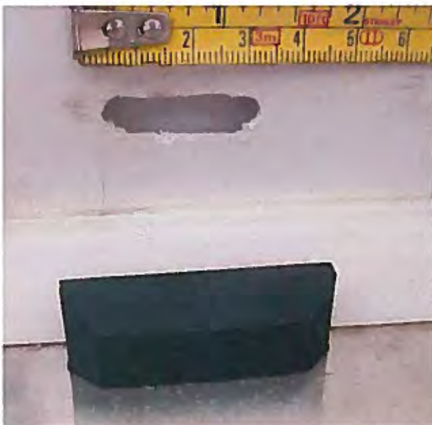
Figure 11 Drainage slot with cover cap removed.
