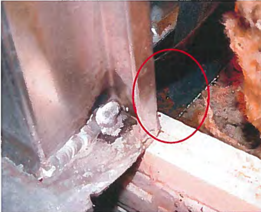
Figure 13 Water on dpc cloak flashing.
