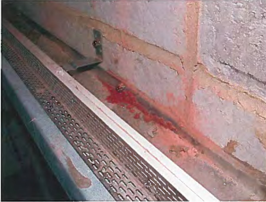
Figure 17 Partially damp debris on surface of flashing that has not transferred to the backing wall.
