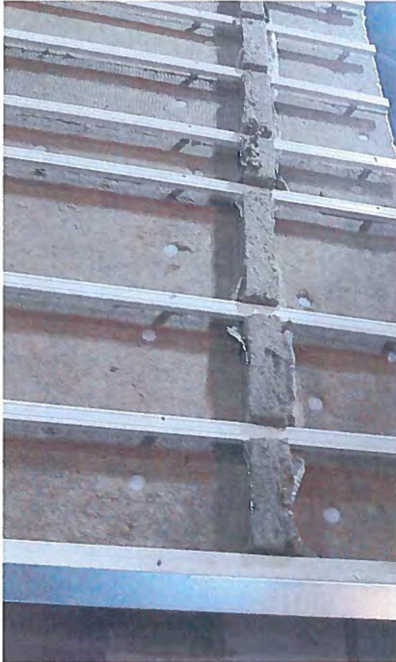
Figure 2. Photograph of the system during construction – insulation layer and vertical fire break with plastic cladding rail penetration.
