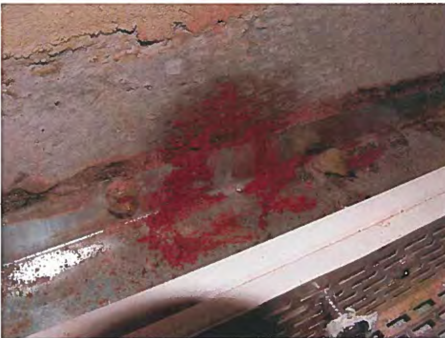
Figure 16 Damp patch on backing wall from water transferred via debris on upper surface of flashing.
