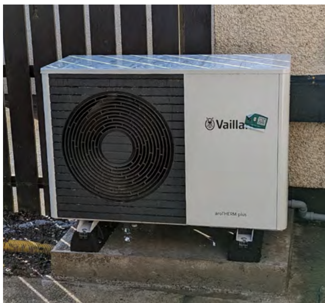
Vaillant Heat Pump as Part of Sunamp Installation
