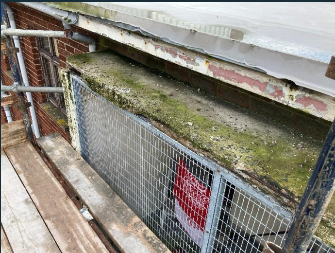
Concrete spalling to balconies.
