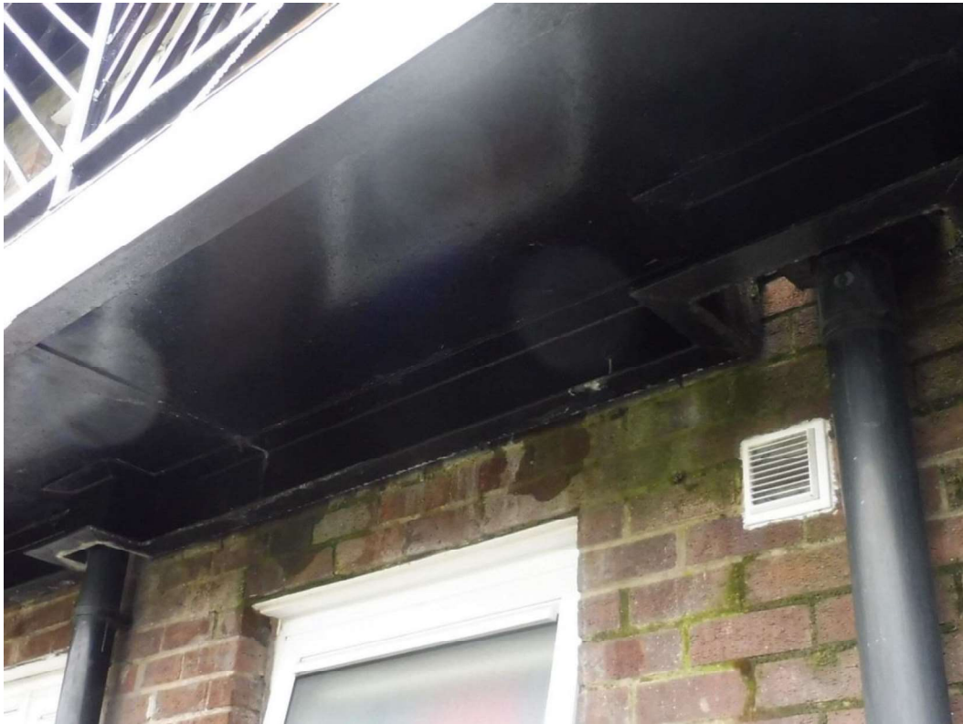
Figure 5 Mould on walls where water runs off balcony and down external walls
