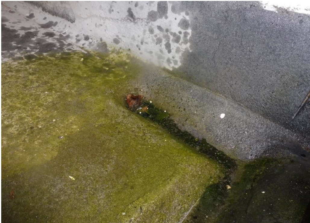
Figure 8 Blocked outlet leading to a 32mm copper pipe
