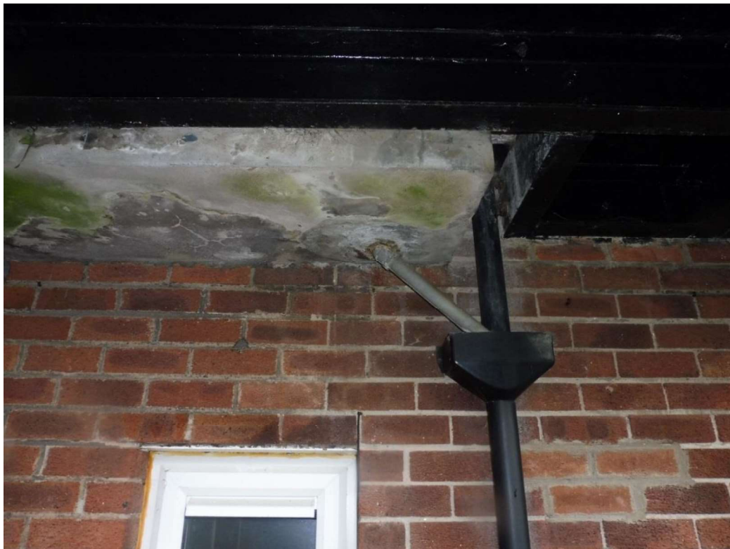
Figure 9 Pipe outlet from drying areas to hopper head
