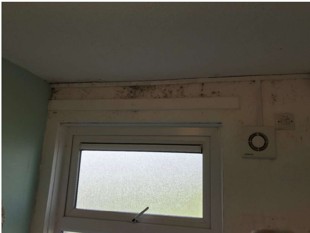
Figure 6 Evidence of water ingress from water coming off balcony to [REDACTED] Glassillan Grove
