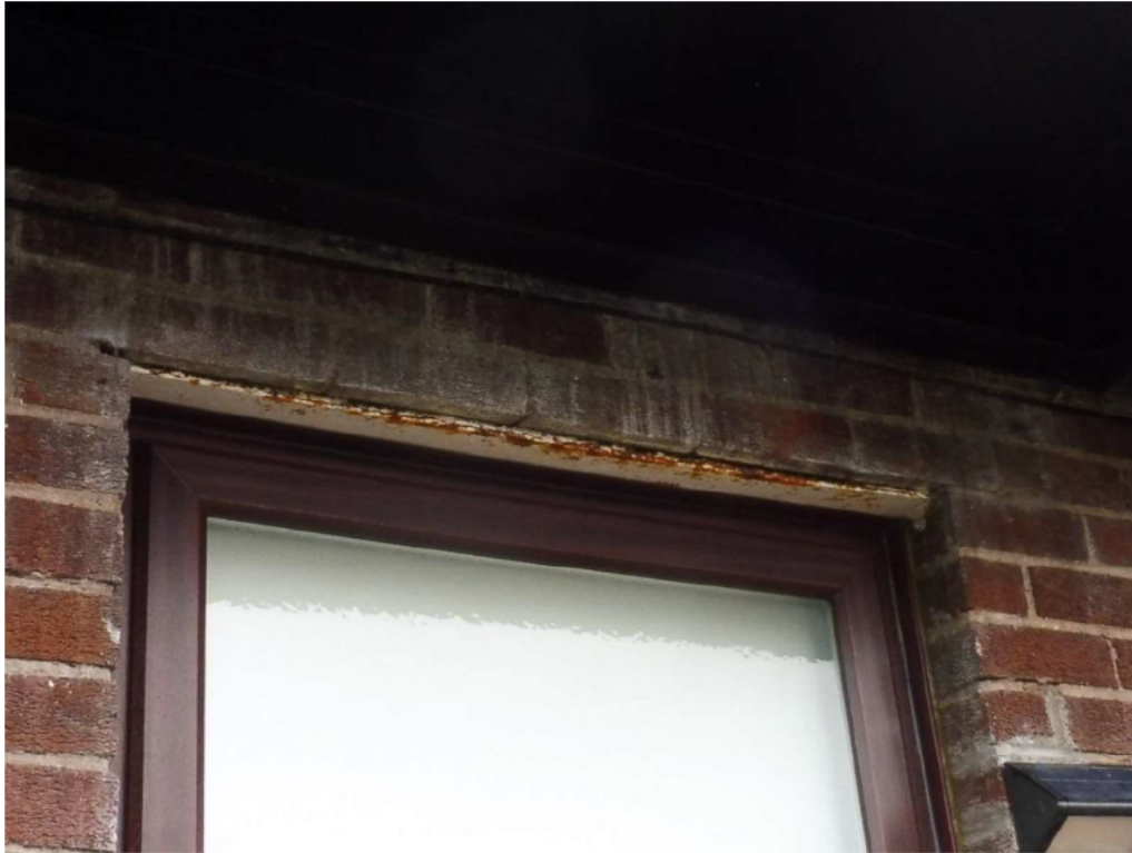
Figure 17 Steel angle irons affected by rust
