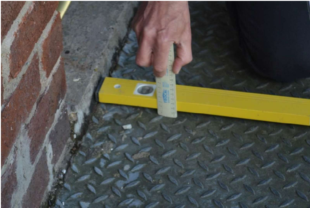
Figure 3 Metal decking laid to incorrect falls into the building
