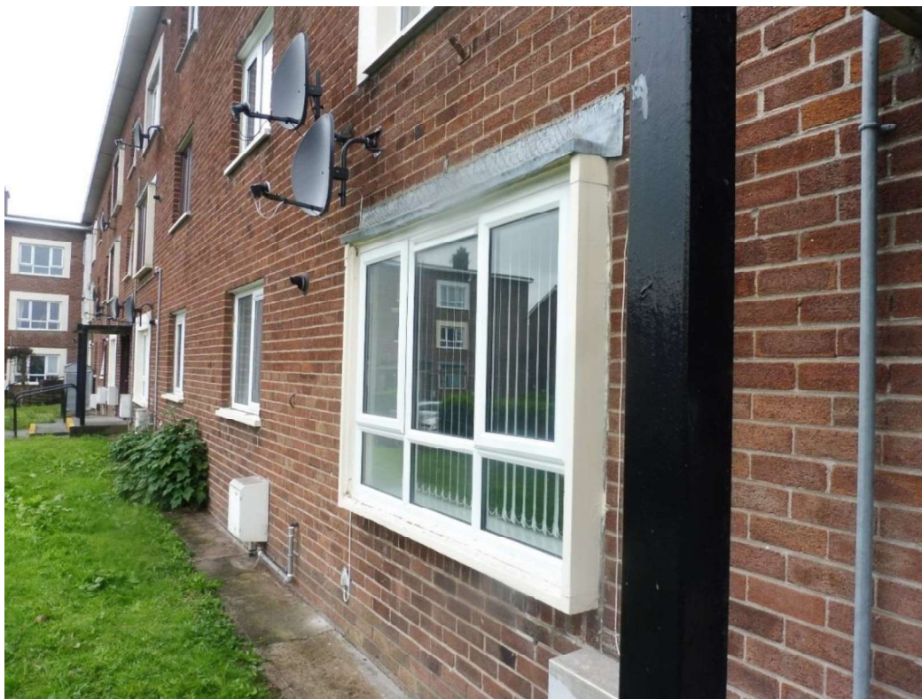
Figure 18 A typical concrete window surround
