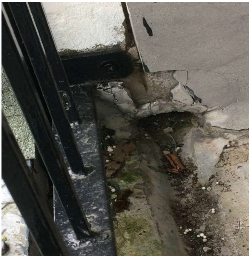
Figure 11 Damage to asphalt possibly leading to water penetration to dwellings below
