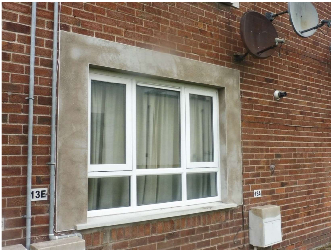
Figure 19 Window where concrete surround has been removed
