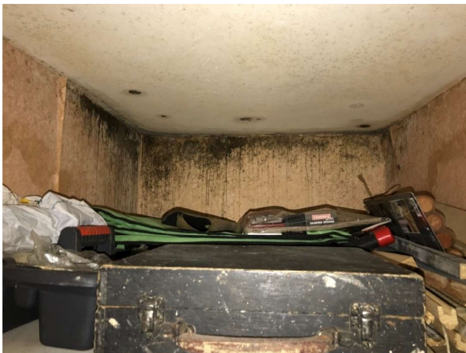
Figure 12 Evidence of water ingress to store below drying area to [REDACTED] Glassillan Grove
