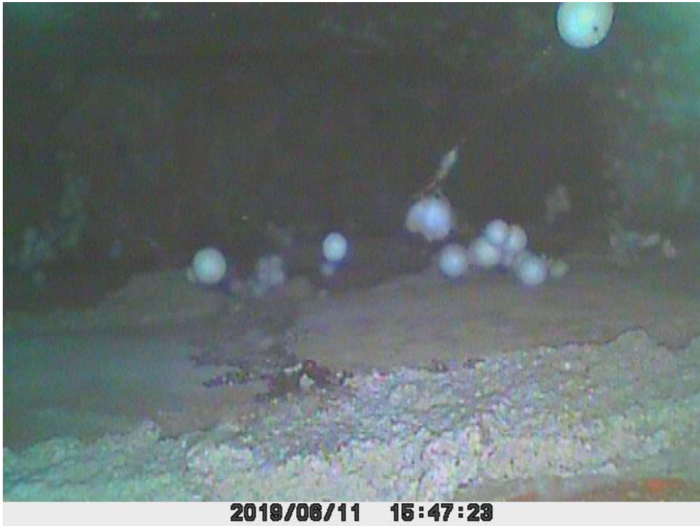
Figure 15 Rossmore Green - Void in insulation
