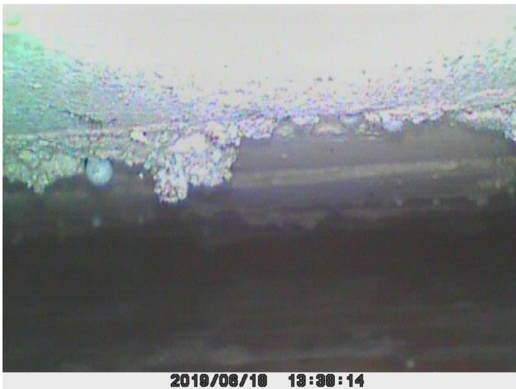
Figure 14 Block [REDACTED] – Glassillan Grove – Insulation absent
