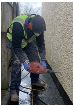
Cavity Wall Insulation Installation
