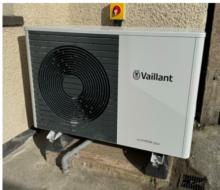
Vaillant Heatpump used in the LCP
