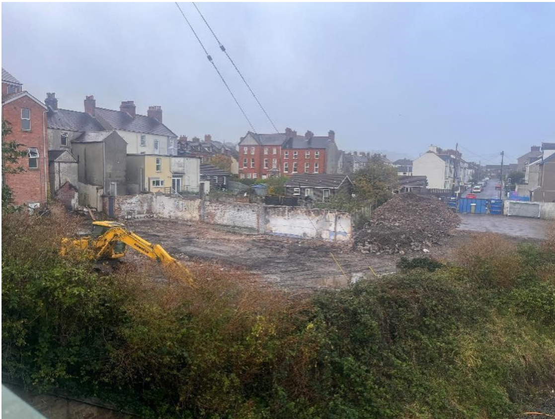
Alpha Housing's new development currently under construction at Windsor Avenue, Whitehead.
