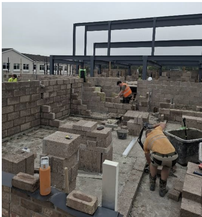
Work underway at Clanmil Housing Association's scheme at Garden Street in Magherafelt. This 19 unit scheme will provide 6 one-bedroom apartments, 6 two-bedroom apartments, 5 two-bedroom houses, one 3-bedroom house and one 2-bedroom wheelchair bungalow
