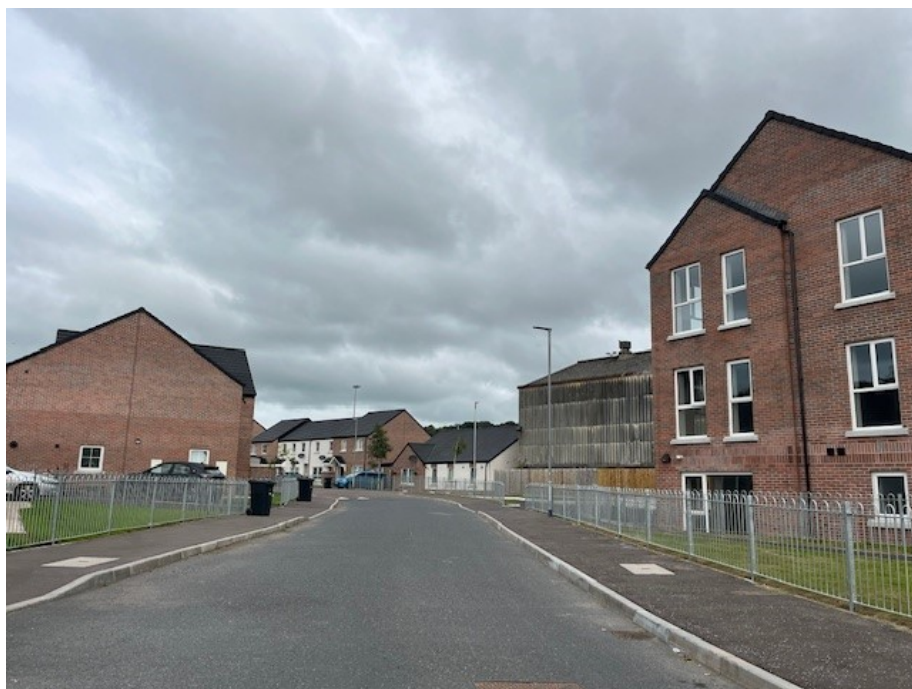
Crannog Way, Dungannon, where Choice Housing Association is currently on site developing a second phase of 27 units, with the following housing mix, 2 one-bedroom apartments, 7 two-bedroom apartments, 6 two-bedroom houses, 7 three-bedroom houses, 2 four-bedroom houses, 2 four-bedroom wheelchair bungalows and 1 three-bedroom wheelchair house.
